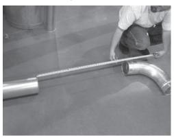
Step 3. Use O-ring to mark cut line and cut.
