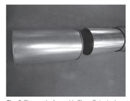
Step 6. Clamp ends of assembly. Clamp O-ring to sleeve.
